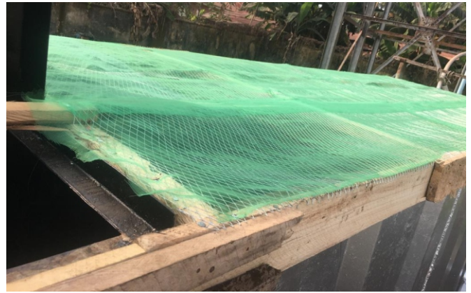
Pictures of work on the filter and tank
