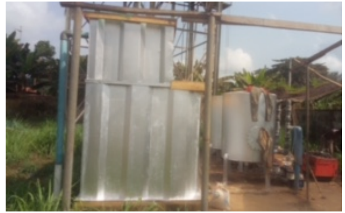
Pictures of the work on the filters, etc
