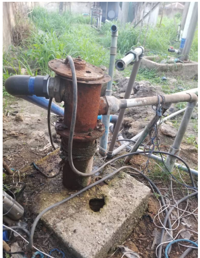
After the repair
