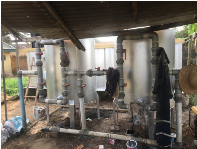
Pictures of the work on the filters, etc
